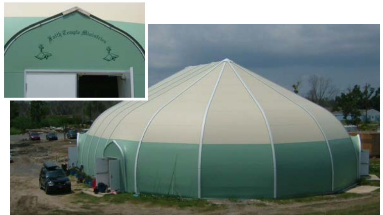
Exterior membrane replaced after Hurricane Katrina.
